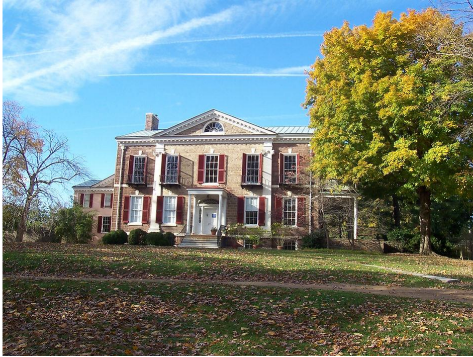
The Highlands Mansion in Fort Washington
