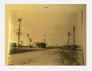
1273 Bethlehem Branch of Reading R. R. Co. Location - Station Ave., Glenside, Poles - P.S.C.G.&E.Co. 40' Span - 114' - P.S.C.G.&E.Co. 2300 V. 3-#4 Primary Street Light 2-#6 Bell Telephone Co. 2 Cross-arms
