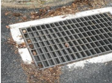
2. Replace storm sewers in the parking lot of the building. This project includes new storm piping and storm inlets. With the paving of the parking areas over the past years, water had been too often routed to the foundation of the building; water now is directed to the storm sewer. This project will protect the building's foundation. Work was done by the Whitpain Public Works staff.
